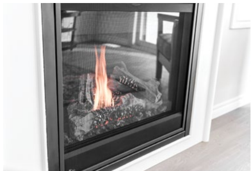
Direct vent gas fireplace (with electronic ignition) with a white mantle finish, as per plan.
