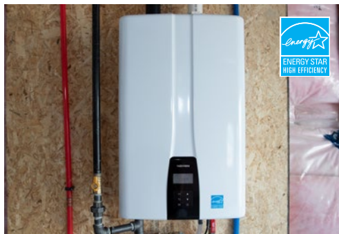
High efficiency hot water tank (rental). Compact in size, these virtually eliminate standby heat loss caused by water sitting in storage style water tanks.
