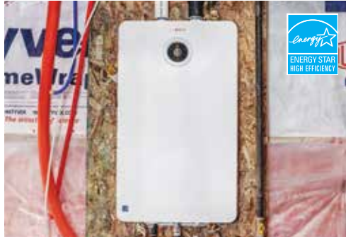
High efficiency hot water tank (not a rental). Compact in size, these virtually eliminate standby heat loss caused by water sitting in storage style water tanks.
